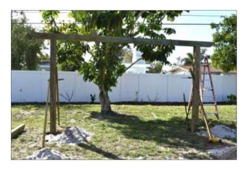
• **Step 12** - If posts are going into footers, fill the holes around the posts with dry concrete. **Do not mix water in the concrete yet**.
