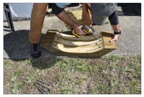
Position the brace with radius cut facing in and flat ends centered on the underside of the beam and side of the post. Make sure the angles are flush to the post and to the top of the rafter, then clamp or have your helper hold the angle in place. Use a hammer to tap both lag bolts to leave an indentation.
