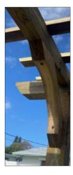
Place the brace back into position so the tip of the lag bolts meet with the pre-drilled holes. Tighten using a 9/16" socket or drill attachment. Repeat for the other post to rafter side angle brace.
