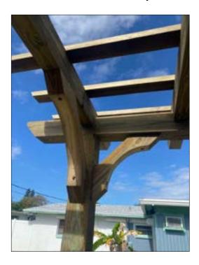
• **Step 20** - Place the top slats into position across the top of the rafters between the marked lines. Ensure each top slat is centered by adjusting for equal measurement outside of the beam on each side (as pictured below). Then screw the top slats down to the rafters using 3" screws provided. Start on one side and make your way across to the other side screwing down the top slats to each rafter.
