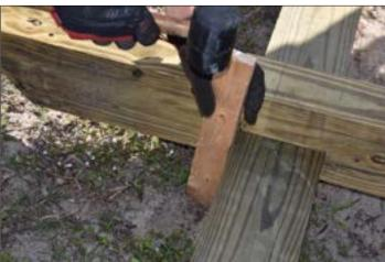
Unscrew and remove the rafters from the beams and move all the boards to the side. Now you should be left with two sets of four marks where the postholes or post bases will be located.
