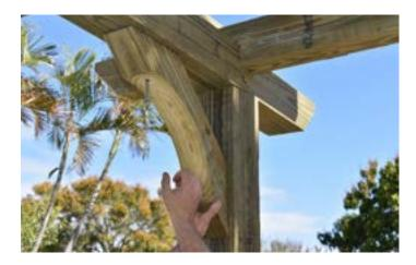
Set the brace aside, and pre-drill holes using a ¼" bit where the indentations are located.
