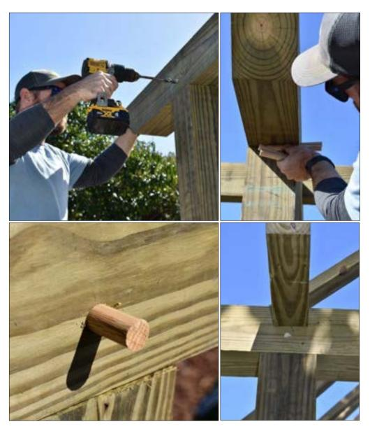
• **Step 18** - Install the remaining rafters over the "X" marks and secure them to the beams with 6" screws through the predrilled holes.
