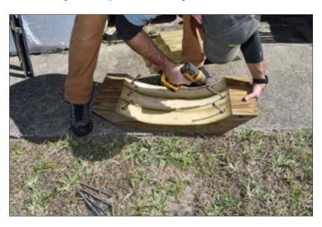
Position the brace with radius cut facing in and flat ends centered on the underside of the beam and side of the post. Make sure the angles are flush to the post and to the top of the beam, then clamp or have your helper hold the angle in place. Use a hammer to tap both lag bolts to leave an indentation.
