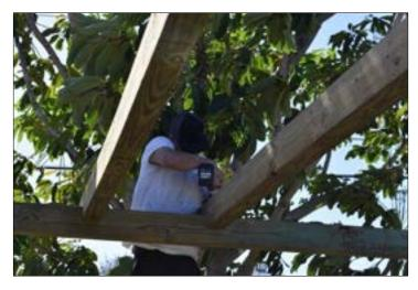
• **Step 19** - Now install the angle braces connecting the post to the outer rafter at each post, securing with 3/8"x6" lag screws provided. Using 9/16" socket or drill attachment, partially screw the lags into the pre-drilled angle braces so about 1/4" of the lag screw tip comes through the brace.
