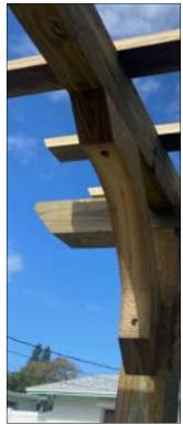
Place the brace back into position so the tip of the lag bolts meet with the pre-drilled holes. Tighten using a 9/16" socket or drill attachment. Repeat for the other post to rafter side angle braces.
