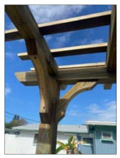
**Step 18** - Place the top slats into position across the top of the rafters between the marked lines. Ensure each top slat is centered by adjusting for equal measurement outside of the beam on each side (as pictured below). Then screw the top slats down to the rafters using 3" screws provided. Start on one side and make your way across to the other side screwing down the top slats to each rafter.
