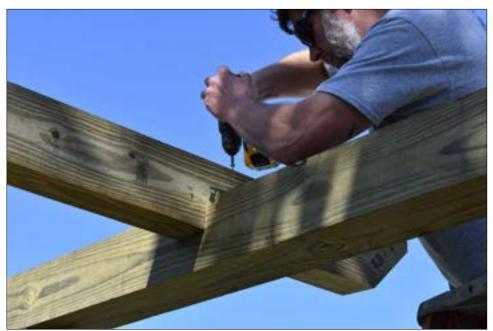
When the first two rafters fit squarely over the beams, secure the rafters to the beams using 6" screws provided through the predrilled holes in the rafter onto the top of the beams.
