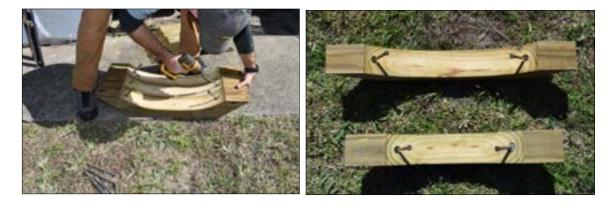
Position the brace with radius cut facing in and flat ends centered on the underside of the beam and side of the post. Make sure the angles are flush to the post and to the top of the rafter, then clamp or have your helper hold the angle in place. Use a hammer to tap both lag bolts to leave an indentation.
