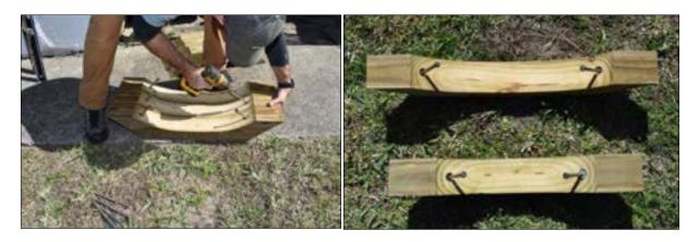
Position the brace with radius cut facing in and flat ends centered on the underside of the beam and side of the post. Make sure the angles are flush to the post and to the top of the beam, then clamp or have your helper hold the angle in place. Use a hammer to tap both lag bolts to leave an indentation.
