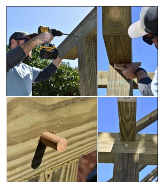
• **Step 15** – Install the remaining rafters over the "X" marks and secure them to the beams with 6" screws through the predrilled holes.
