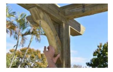
Set the brace aside, and pre-drill holes using a 1/4" bit where the indentations are located.
